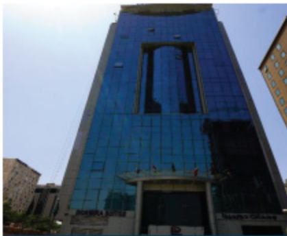
DORMERA HOTEL , RIYADH SUPPLY & INSTALLATION MONDRAIL SYSTEM
