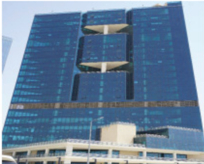
SMASCO TOWER ,RIYADH SUPPLY & INSTALLATION MONDRAIL SYSTEM
