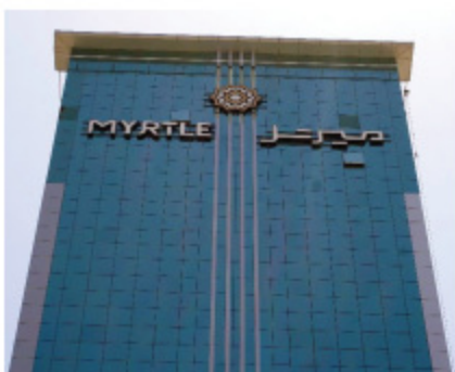
MYRTLE HOTEL , RIYADH SUPPLY & INSTALLATION MONDRAIL SYSTEM
