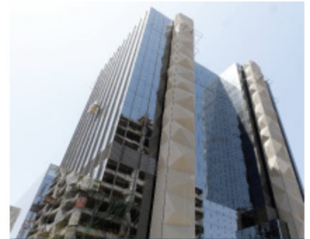
VERONA , RIYADH SUPPLY & INSTALLATION MONDRAIL SYSTEM
