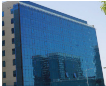
EBDAAT-1 , RIYADH SUPPLY & INSTALLATION MONDRAIL SYSTEM
