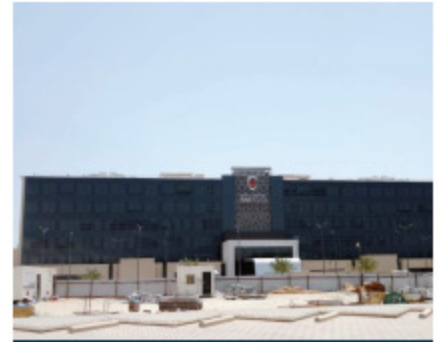
CALLAH HOSPITAL , RIYADH SUPPLY & INSTALLATION MONDRAIL SYSTEM
