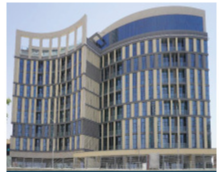
JARIR REAL STATE , RIYADH SUPPLY & INSTALLATION MONDRAIL SYSTEM
