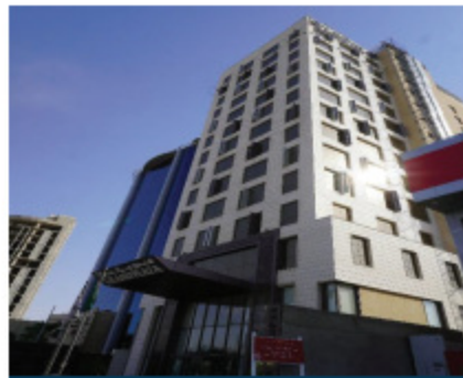
GRAND PLAZA , RIYADH SUPPLY & INSTALLATION MONDRAIL SYSTEM
