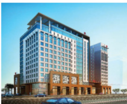
ALESAYI PLAZA, JEDDAH SUPPLY & INSTALLATION MONDRAIL SYSTEM
