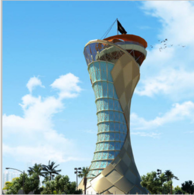
ARAR WATER TANK
