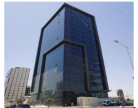
EMAAR AL MADEN-5 SUPPLY & INSTALLATION MONDRAIL SYSTEM
