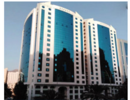
8 BUILDINGS , MAKKAH SUPPLY & INSTALLATION MONDRAIL SYSTEM
