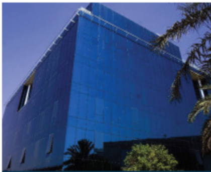
TOURISM AUTHORITY , RIYADH SUPPLY & INSTALLATION MONDRAIL SYSTEM
