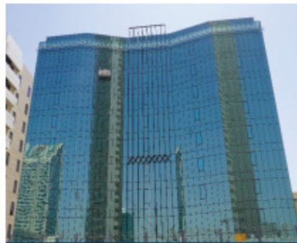
EBDAAT-3 SUPPLY & INSTALLATION MONDRAIL SYSTEM
