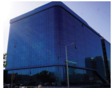
EBDAAT-2 , RIYADH SUPPLY & INSTALLATION MONDRAIL SYSTEM
