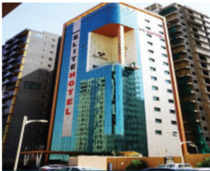
ELITE HOTEL , RIYADH SUPPLY & INSTALLATION MONDRAIL SYSTEM
